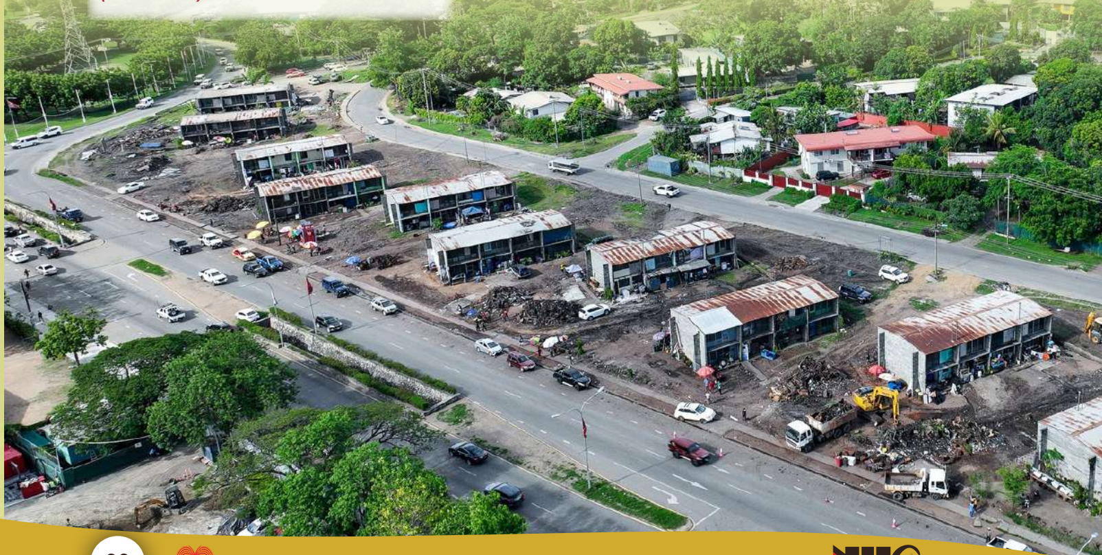
The run down NHC facility for upgrade (5mile NCD)
